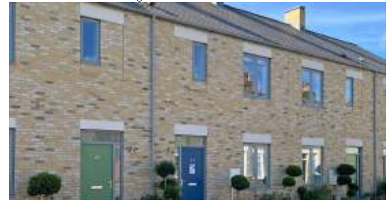
Flat fronted terrace with stone detailing
