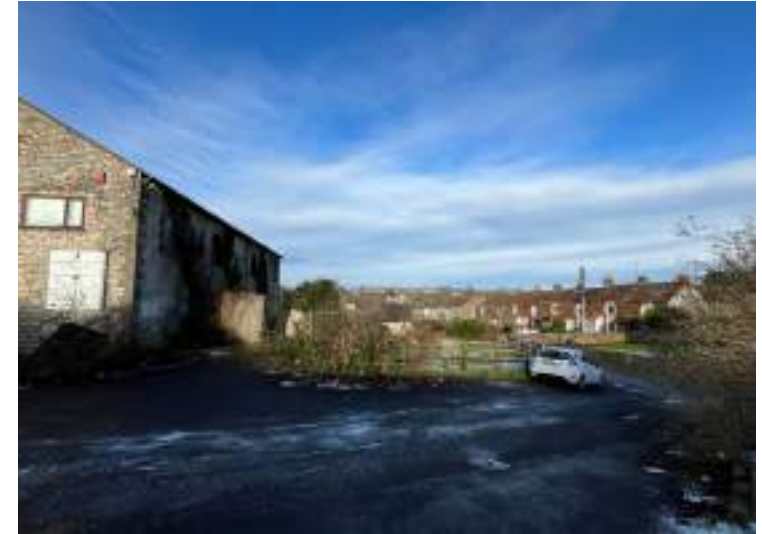
View east of existing Gasworks building with terraced housing behind
