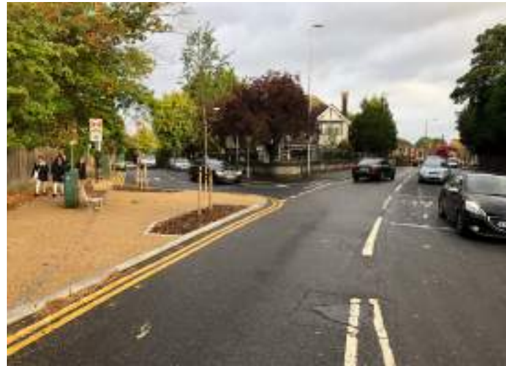
The same junction as shown above after being modified to narrow the carriageway and create a safer pedestrian place
