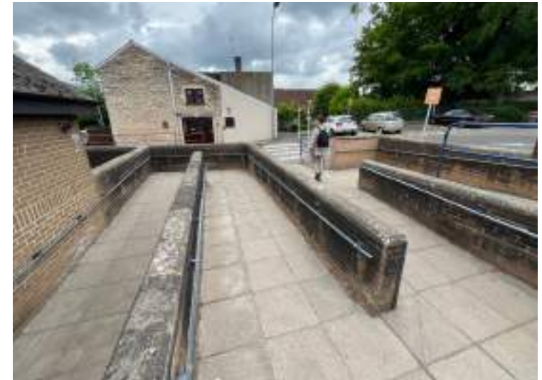
The pedestrian ramps from the Sainsbury's store to the car park are narrow and unnecessarily complicated
