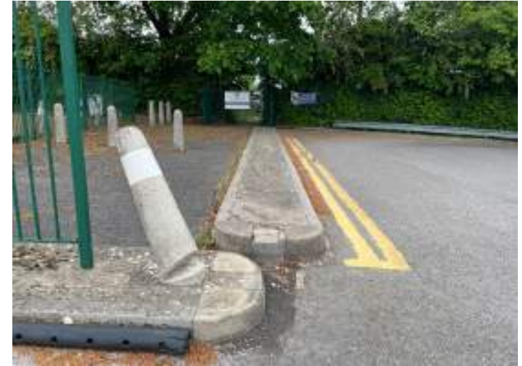
The existing school entrance which is accessed from the car park on the north east side
