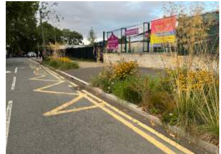
SUDS planting used to create a buffer between pedestrians and vehicles outside a primary school
