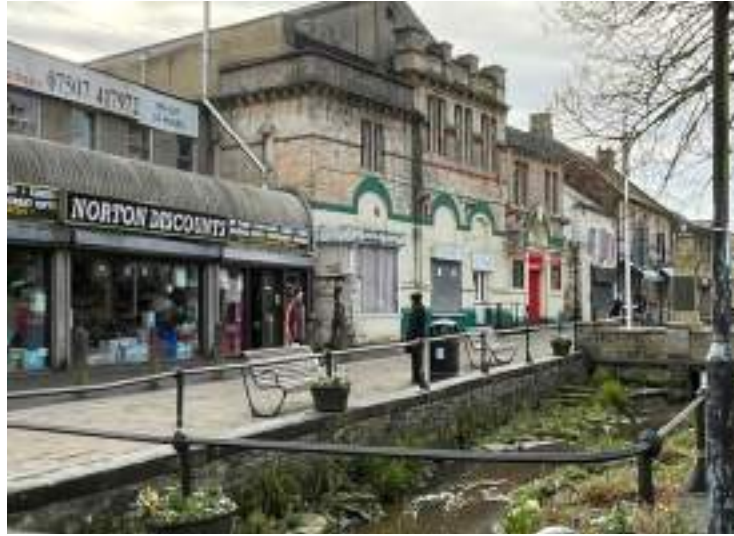
The existing building today - comparison with the historic photo demonstrates the extent of changes including to the roof
