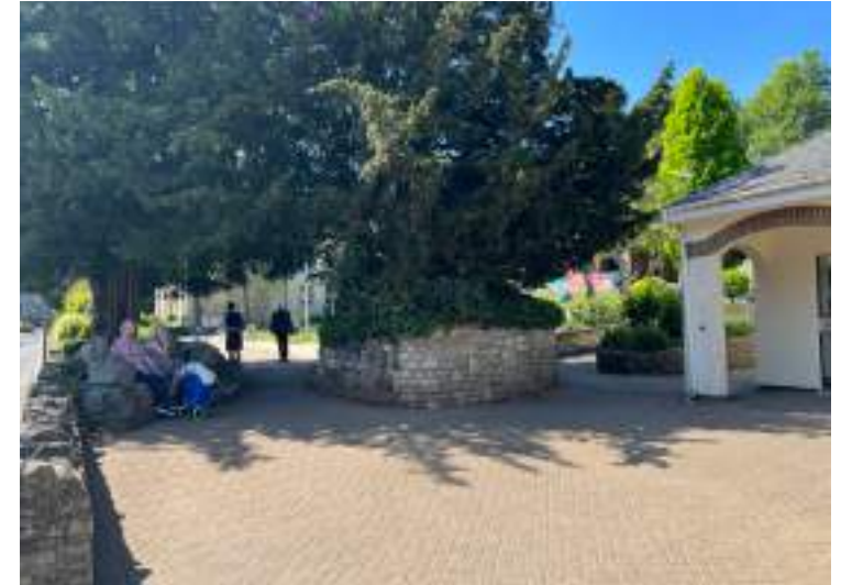
A fragment of historic grotto wall exists in the south east corner of the gardens, but is a barrier to movement and legibility
