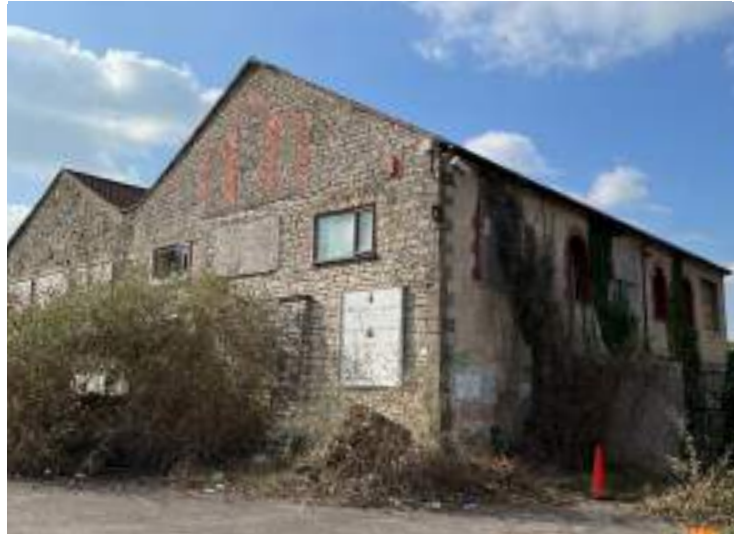
View east of existing Gasworks building
