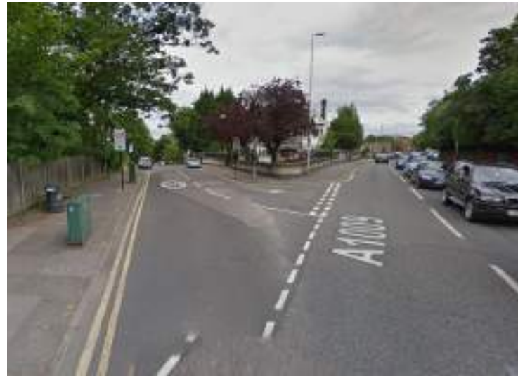
An example of a wide bell-mouth at a junction built to dated highway design standards with a very long pedestrian crossing
