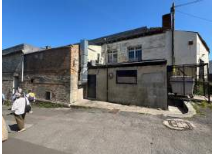
Layers of accretions which could usefully be removed to establish a sound basis for refurbishment
