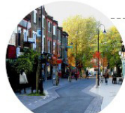
London, UK: Reimagined carriageway within the Core High Street creating a safer environment for people walking & cycling. Integrating street planting with seating to create spaces for rest.
