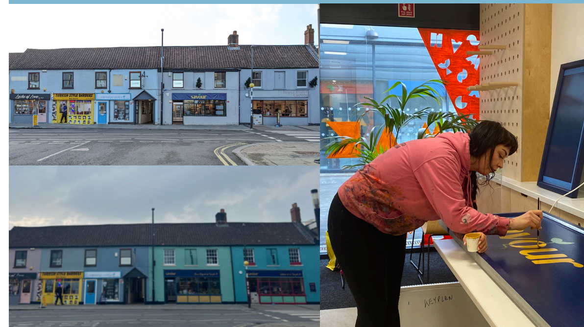
Left: 20-30 Temple Street before and after shop front improvements
