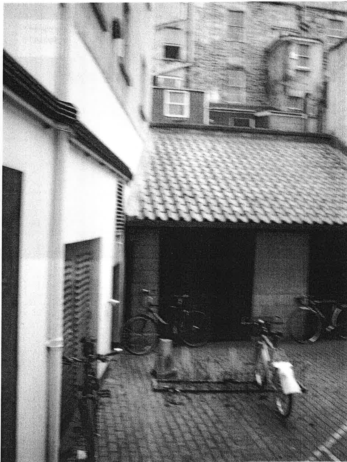
Photo3: showing height of drop from perimeter wall to IPL courtyard and access to internal areas of the premises
