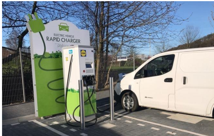
Figure B-3: Rapid charging point
