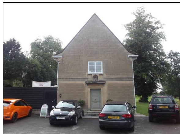
West elevation of 1 Alice park
