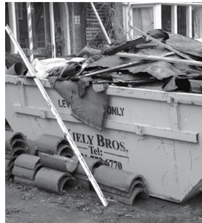
Segregating waste onsite for recycling
