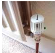
Install heating controls
