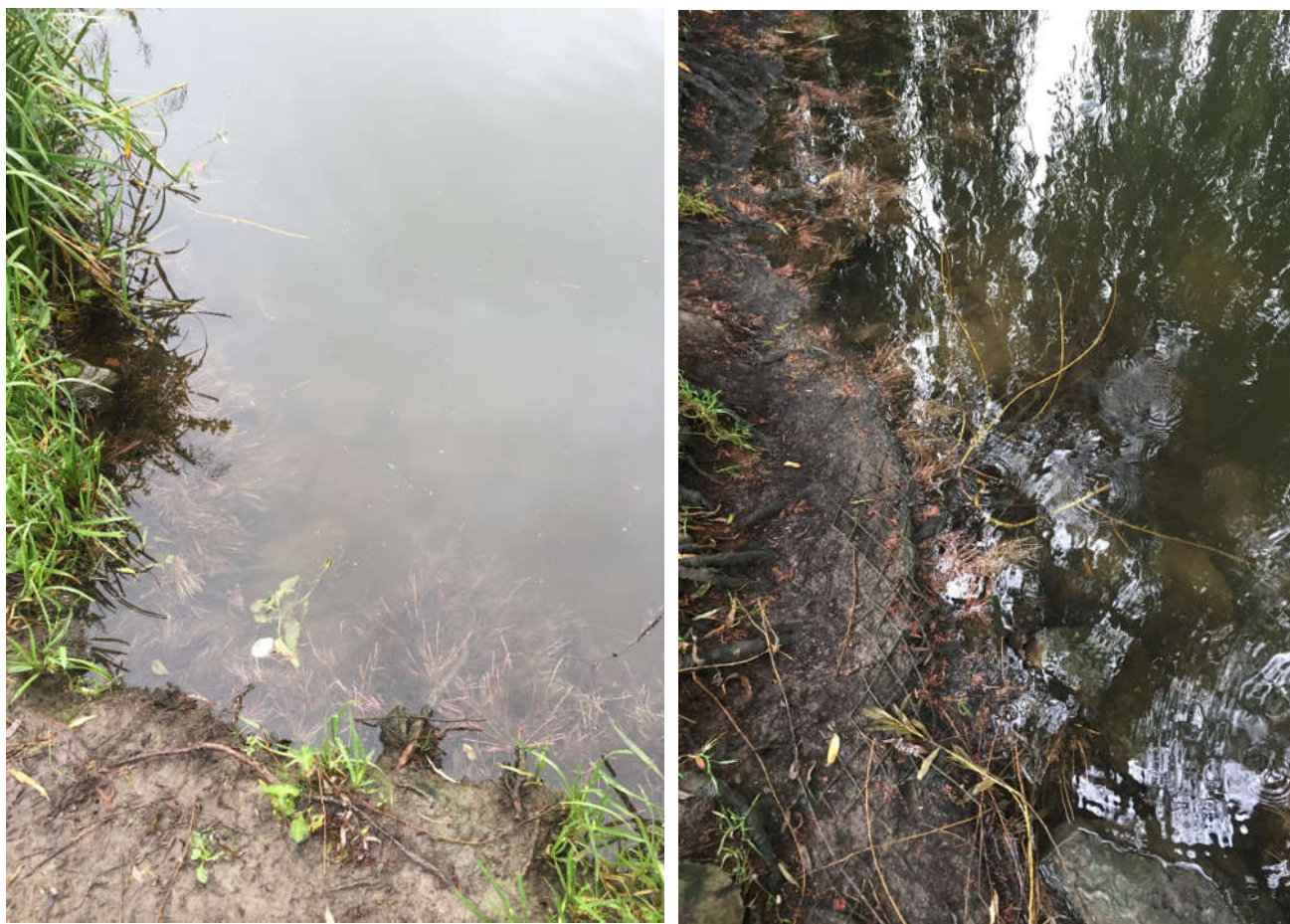
Figure 4-9 - Rock revetment (left) and exposed coir roll (right)
