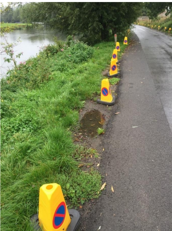
Figure C-7: Damage to verge
