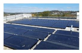
224 photo voltaic panels have been installed, which cover an area half the size of a five-a-side football pitch, on the new office development at Bath Quays South. The development now hosts the largest solar array in Bath and will provide the building with a reliable source of renewable energy.
