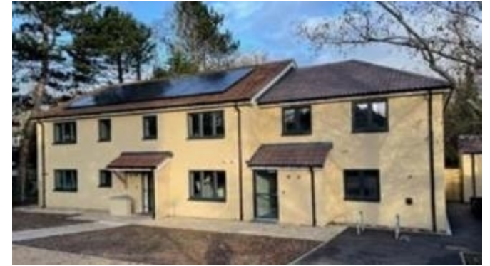
Theobald House, designed to Passivhaus standard.
