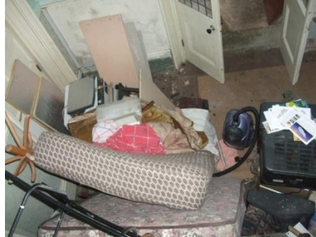
Ground Floor hallway
