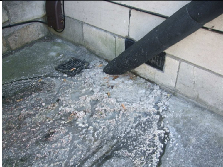
Blocked front drain
