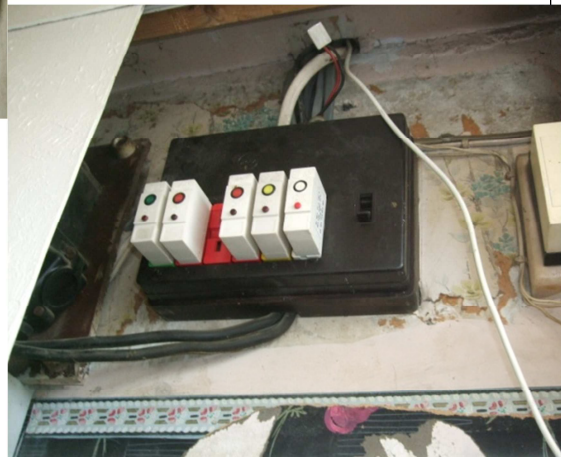
Fuse board, dated and no earthing
