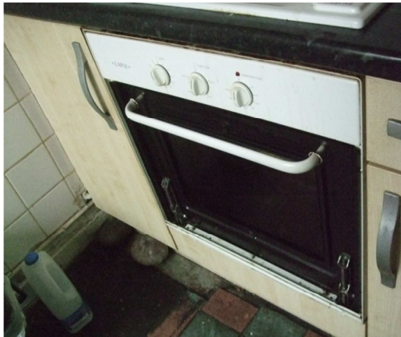
Front panel missing off oven
