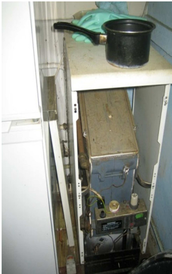
Damaged boiler with front panel missing
