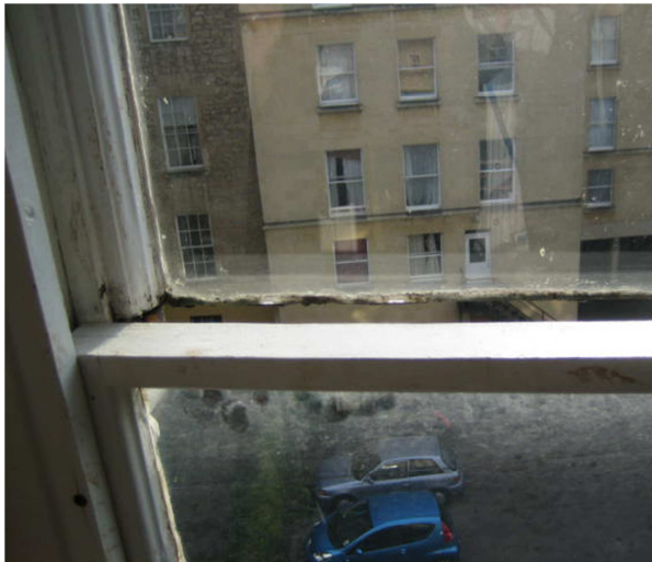
Broken sash window
