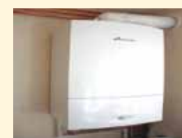
gas condensing boiler
