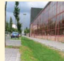
create swales to hold the rainwater
